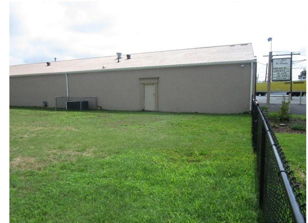
A rain garden can be installed southwest of the building to capture, treat, and infiltrate stormwater runoff from the roof. Downspout planter boxes can be constructed and installed at each of the four downspouts on the east side of the building to capture and treat the stormwater runoff from the rooftop. A preliminary soil assessment suggests that more soil testing would be required before determining the soil's suitability for green infrastructure.
