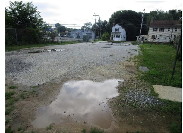
Parking spaces in the parking lot to the northeast side of the building can be converted to porous pavement to capture and infiltrate stormwater runoff from the parking lot. A preliminary soil assessment suggests that more soil testing would be required before determining the soil's suitability for green infrastructure.
